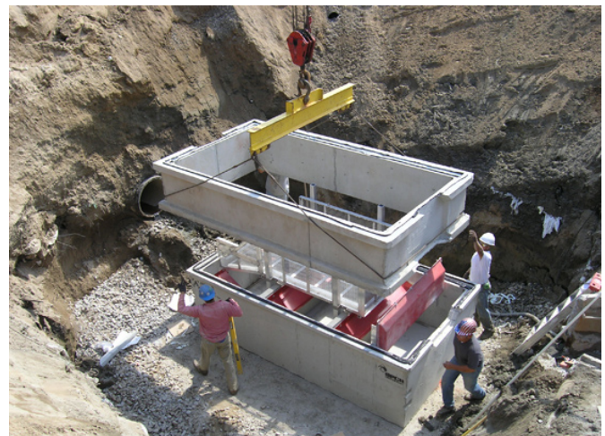
First mid-section being lowered into position
