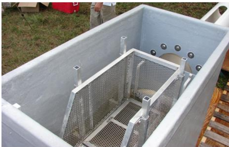
Figure 1 - Sieve strainer screen of Type 2 baffle box
