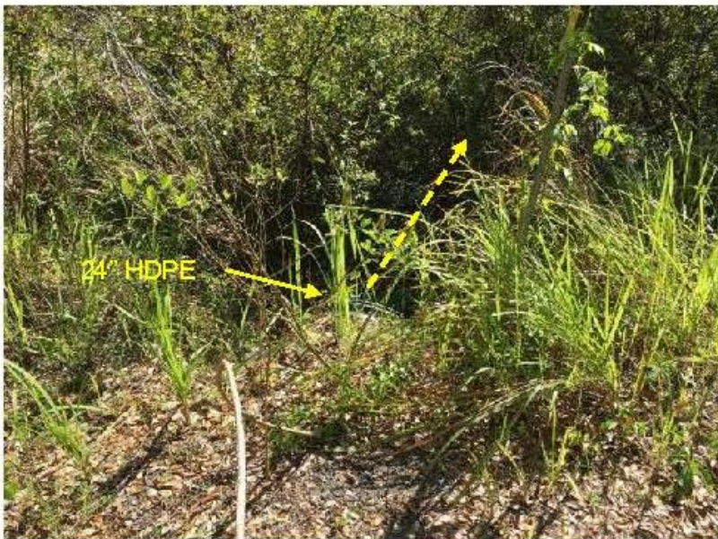
Outfall discharge through berm
