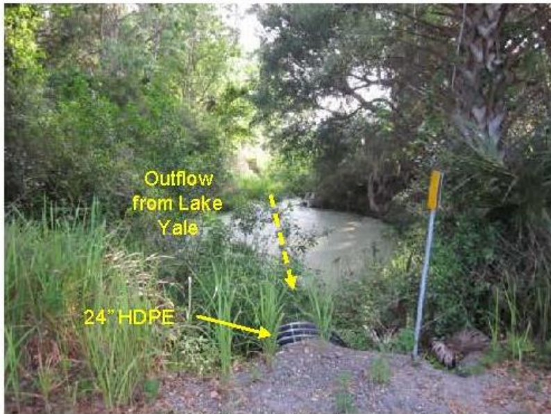
Lake Yale outfall structure
