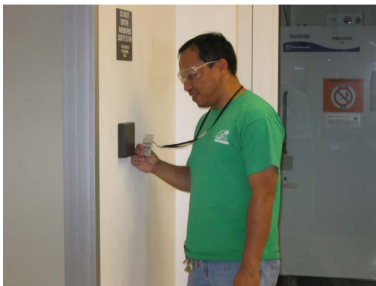
Figure 2: Proximity Readers provide access to restricted areas within the facility with an authorized proximity card.
