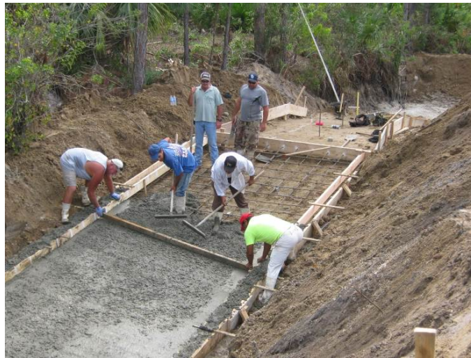
FIGURE 4: BREVARD COUNTY VALKARIA LAKES PROJECT UNDER CONSTRUCTION
