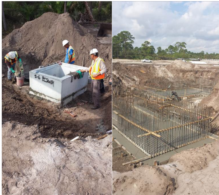
FIGURE 5: INDIAN RIVER COUNTY PC SOUTH (OSPREY MARSH) NUTRIENT REMOVAL FACILITY UNDER CONSTRUCTION
