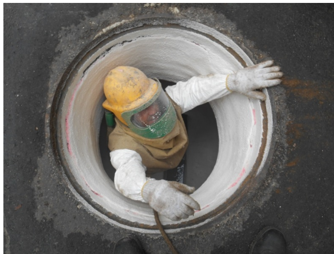
FIGURE 2: CITY OF ATLANTIC BEACH MANHOLE REHABILITATION
