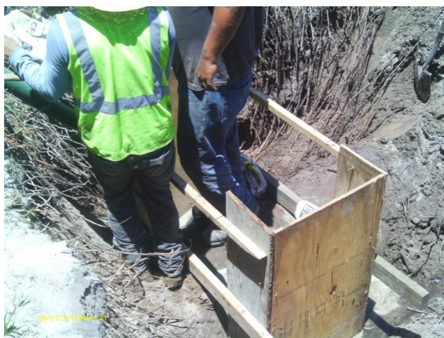
FIGURE 8: TOWN OF SEWALL'S POINT INDIALUCIE PROJECT UNDER CONSTRUCTION
