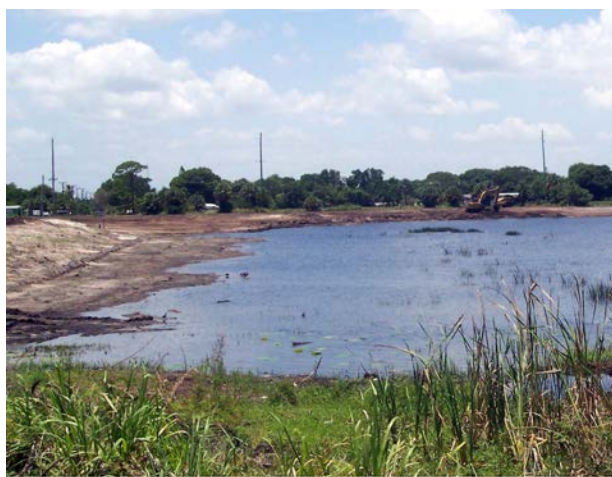
Indian Hills Recreation Area Stormwater Improvements - Lake Expansion - 06/26/14
