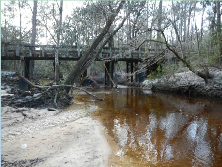
Scott Road Bridge, looking downstream. Access the stream from the east side of the bridge (to the right)
