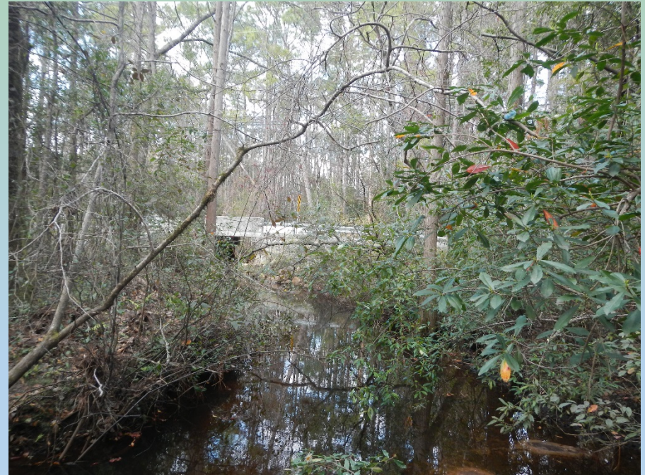
Looking downstream at the Alva Thomas bridge, from the 0 m mark
