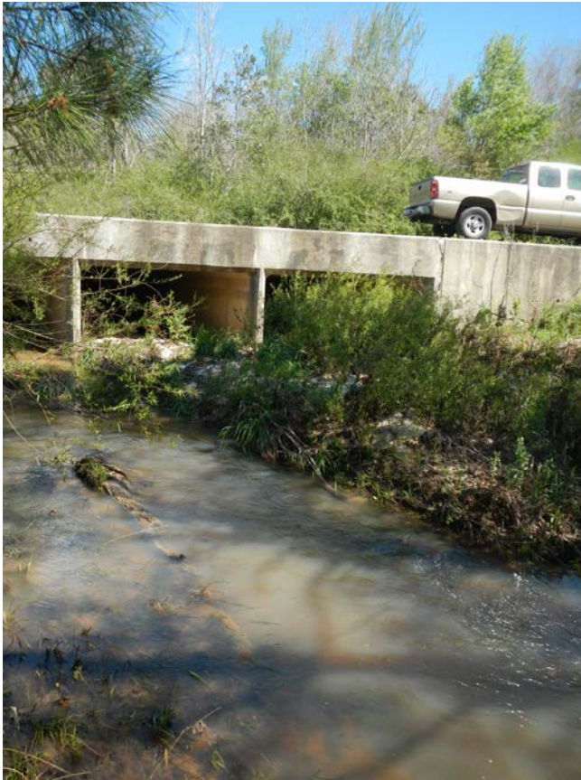
Site is upstream of bridge.
