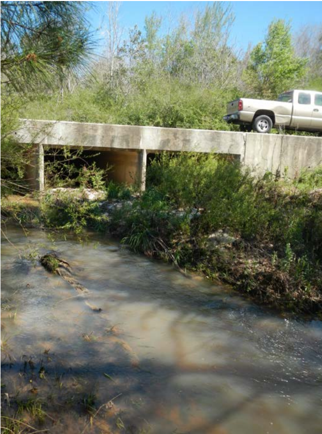
Site is upstream of bridge.
