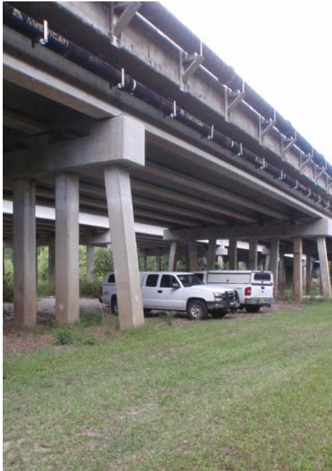
Park under bridge
