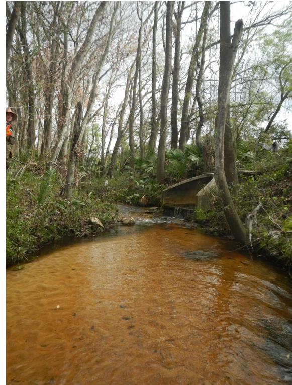
Looking downstream near the 100 m mark
