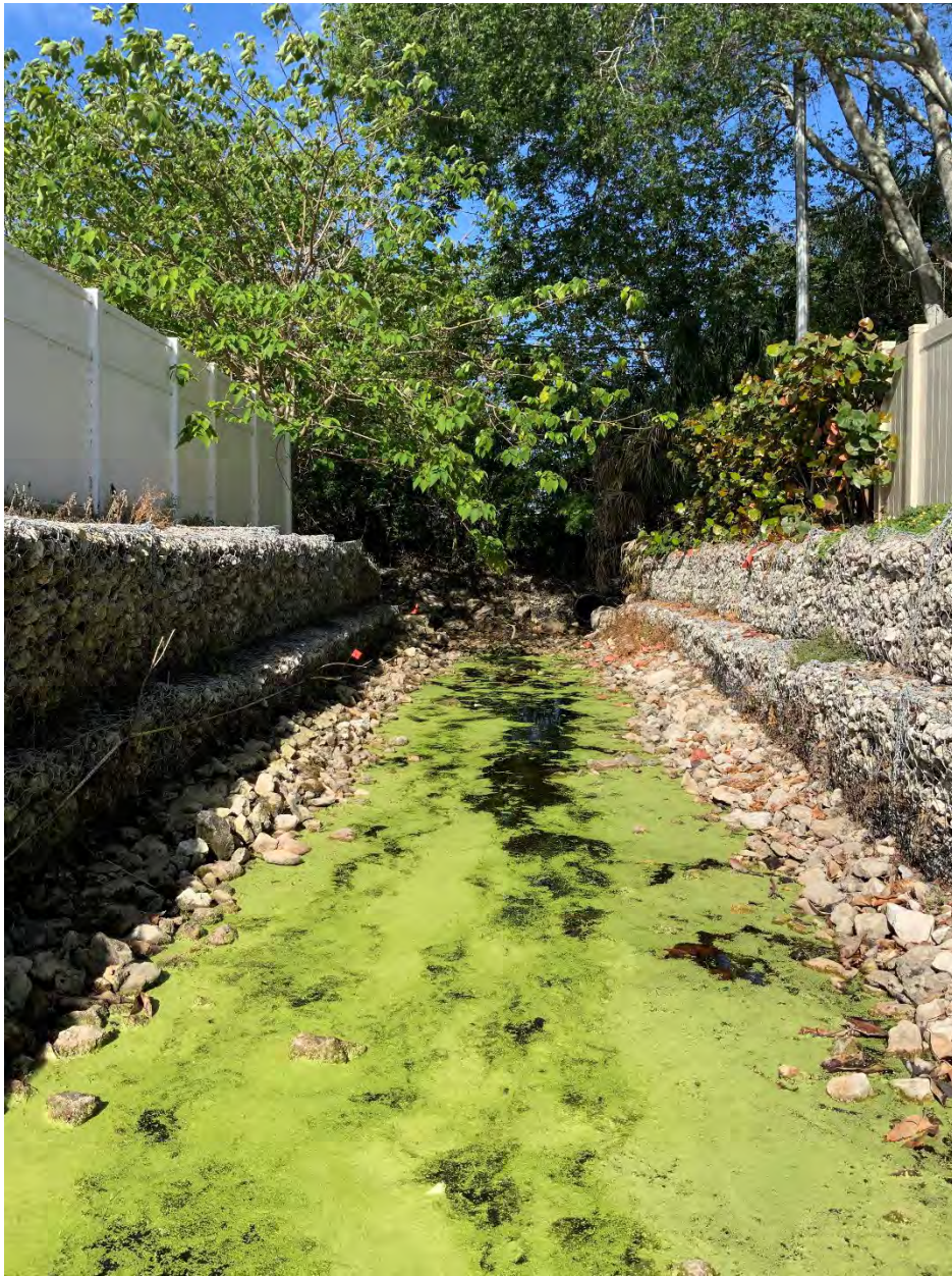
Channel E same location as above, just looking west (confluence of Channel C is at end)
