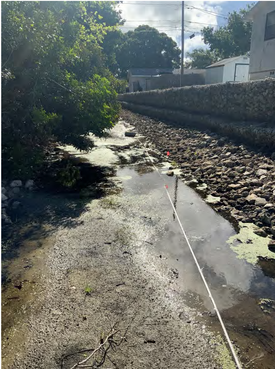
Channel E looking east (28.027145 N, -82.777056 W).
