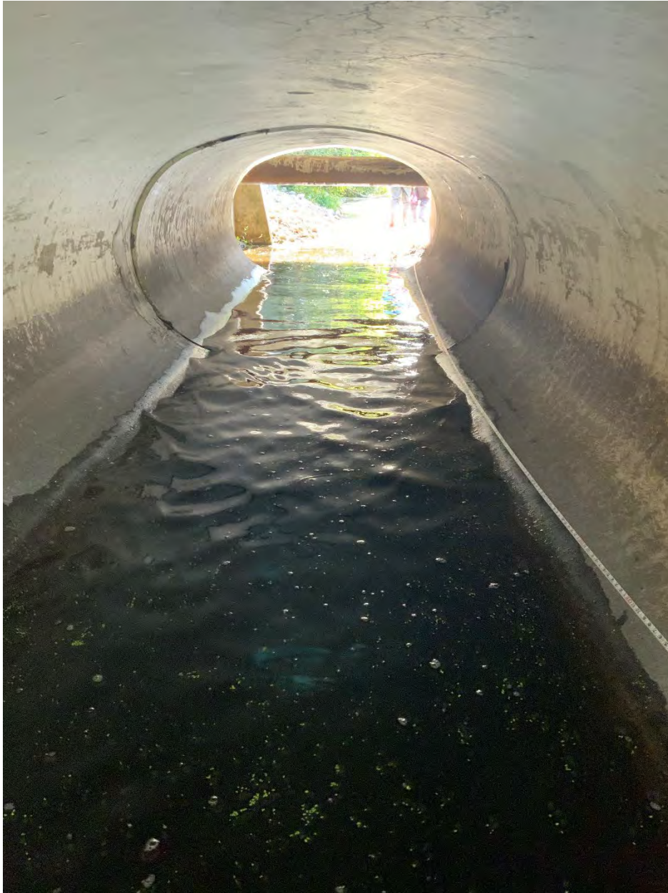
Channel E looking east, under St Catherine Dr W (28.027151 N, -82.777315 W).
