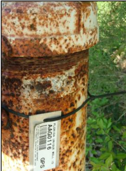
Figure 35. Well with a FLUWID tag.
