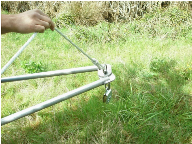
Figure 4. Bowline Knot Used to Attach the Bi-pod Extension Top.
