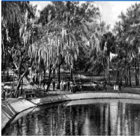
Figure 2-2A. Photograph from 1908 showing the concrete rim enclosing the Sulphur Springs Pool.
