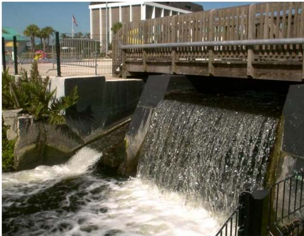
Figure 2-4. Discharge structure at Sulphur Springs Pool.
