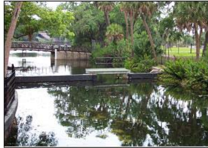
Figure 2-6B. Weir with opening extending across Sulphur Springs Run, showing the footbridge at the mouth of the spring run in the background.
