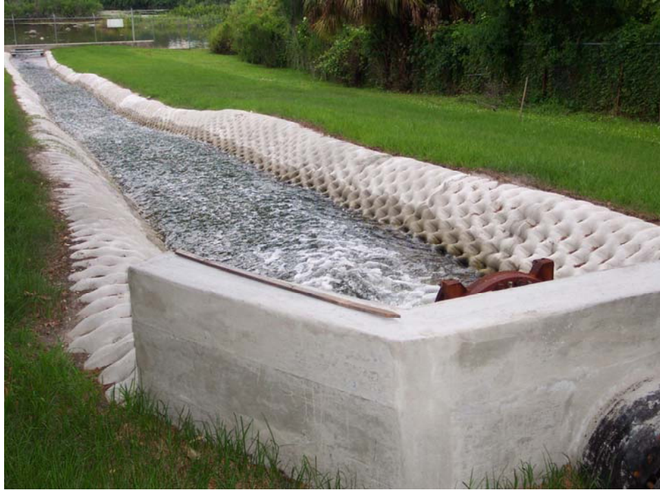
Figure 2-13. Flume discharge structure at base of reservoir dam.
