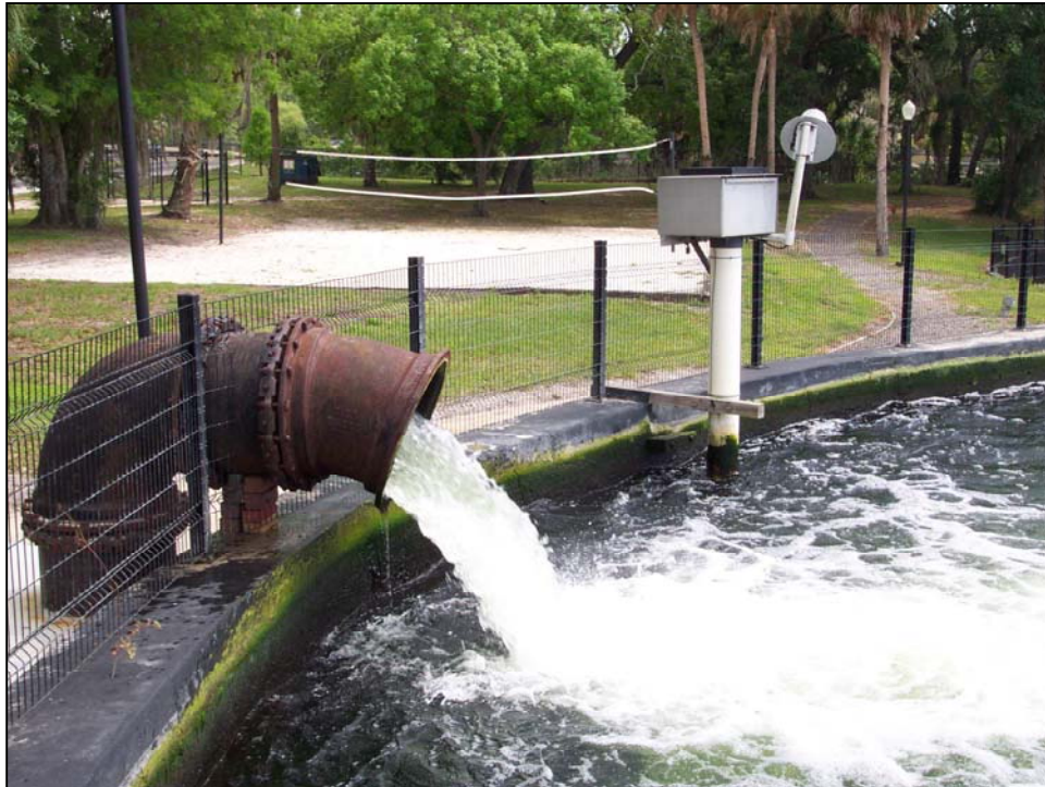
Figure 2-14. Return flow structure at Sulphur Springs Pool.
