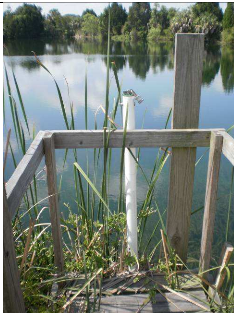
Photograph 8 – View of monitor well located on subject Property.
