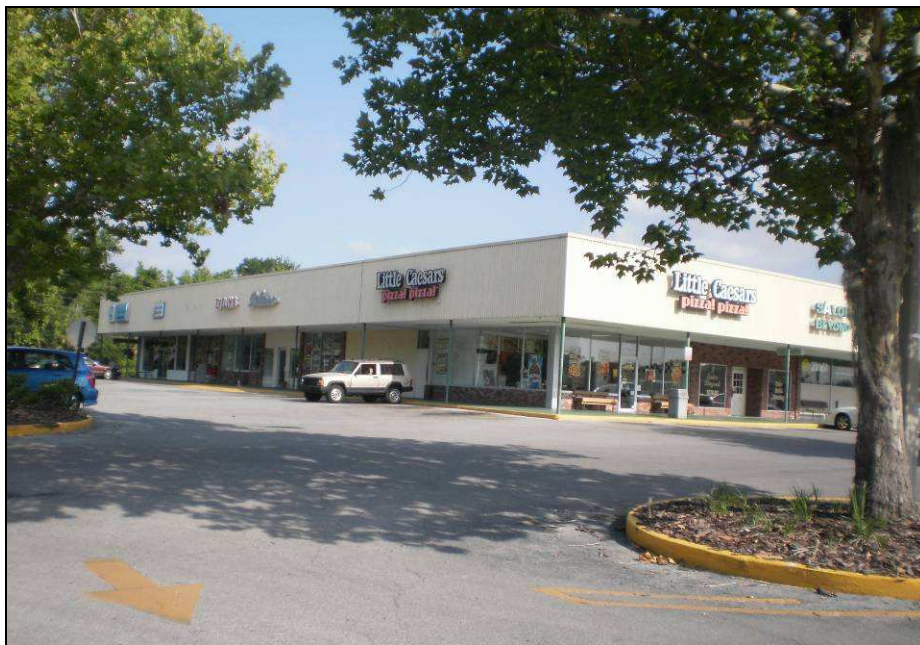
Photograph 12 – View of northeastern adjacent property.
