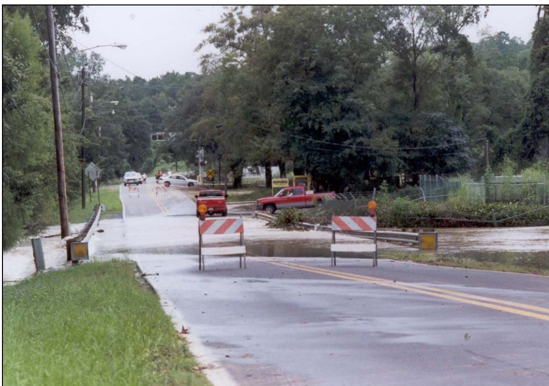
Figure 5.1.4: Weems Pond flooding into Upper Lake Lafayette, summer 2002. This flooding is from Tropical Storm Helene. The storm water is not getting much treatment here.
