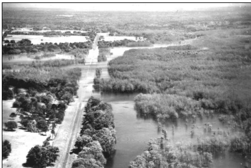
Figure 5.1.6: Flood damage on the track of the Seaboard Line that divides Alford Arm from Lower Lake Lafayette (April 2, 1948)
