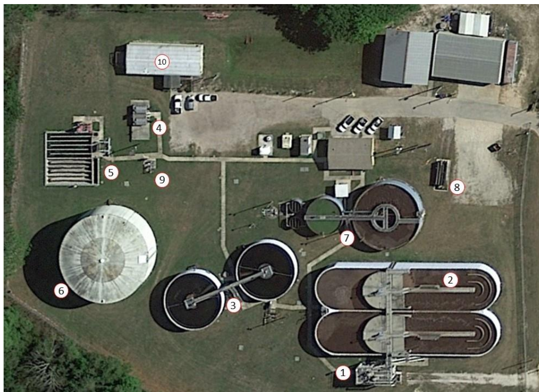
Figure 3-9: Sampey WWTP Aerial View
