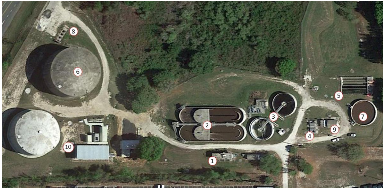
Figure 3-10: Sunshine WWTP Aerial View
