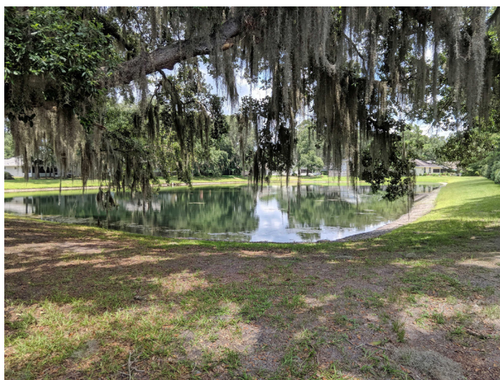
Figure 1. A typical stormwater pond in a Florida community. Note the bank erosion and lack of plantings along its perimeter.
