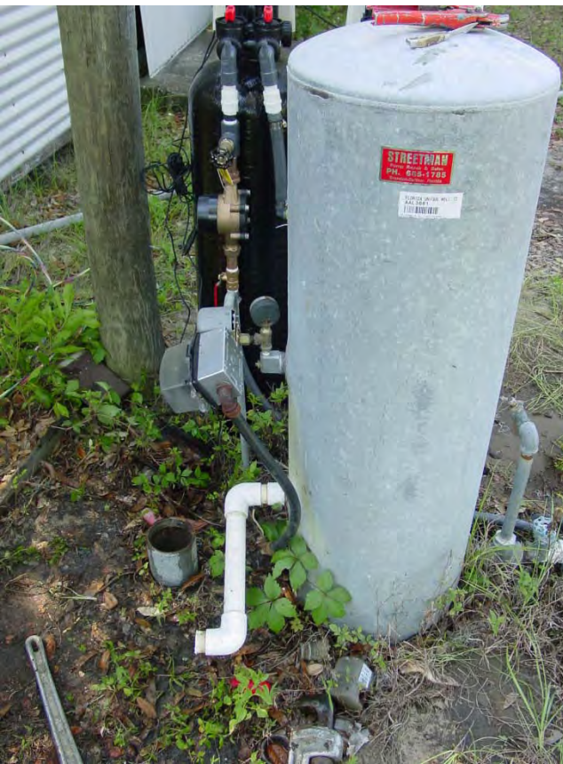
Typical Private Supply Wells with Pressure Tanks
