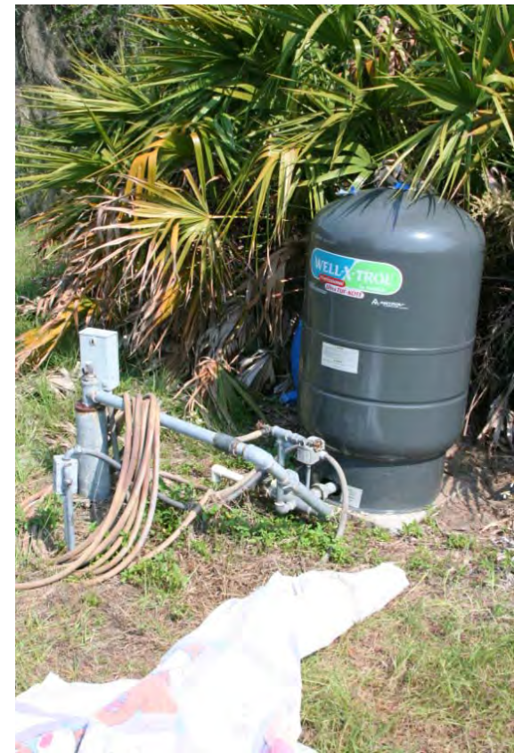
Typical Private Supply Wells with Pressure Tanks
