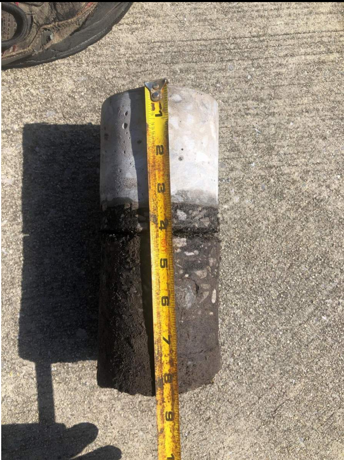
Core P-8 - Approximately 3 1/4 Inches of Cementitious Concrete & 5 Inches of Asphaltic Concrete
