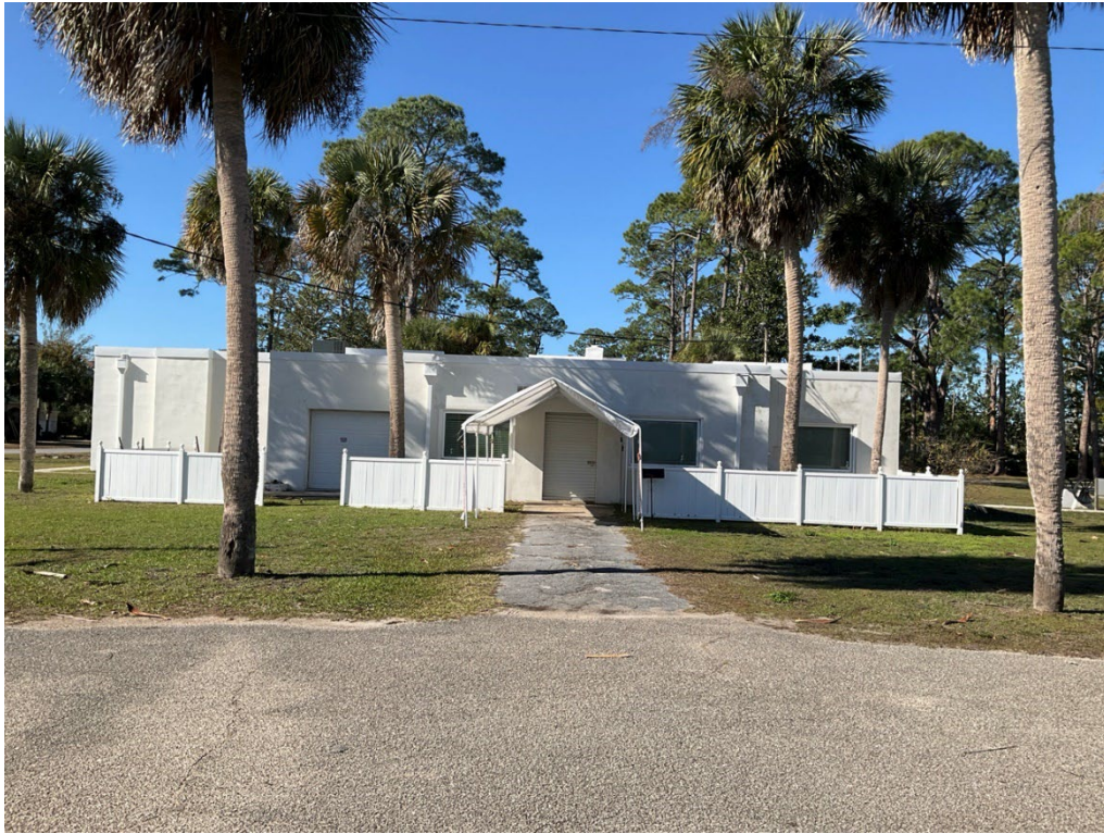
Figure 6-5. Photograph of 8GU00228 – 4, facing west.
