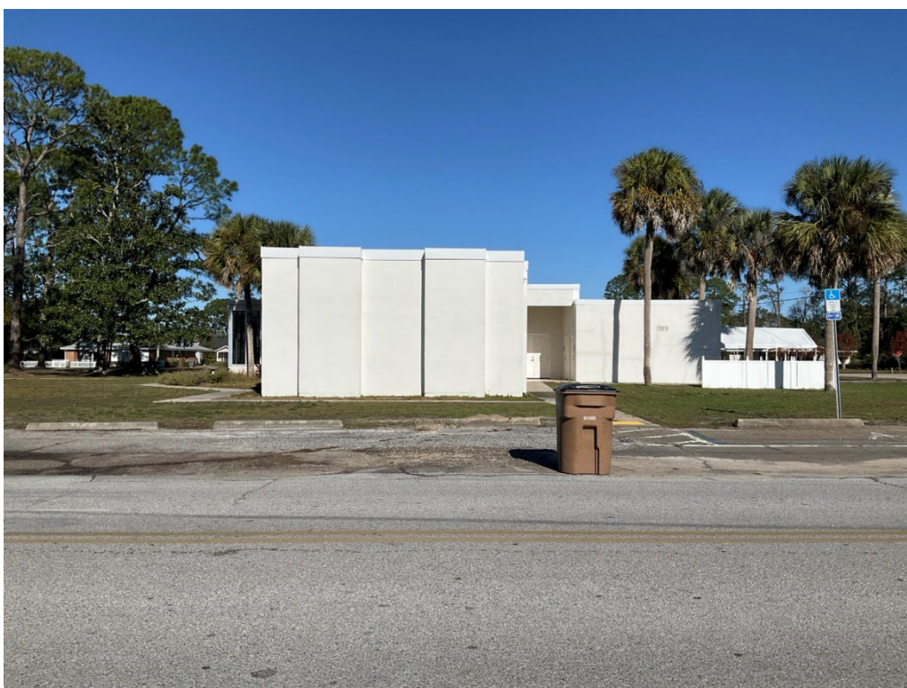
Figure 6-4. Photograph of 8GU00228 - 3, facing north.
