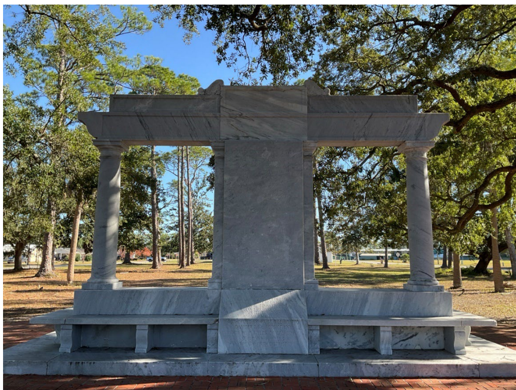
Figure 6-8. Photograph of 8GU00230 – 2 (monument rear), facing east.
