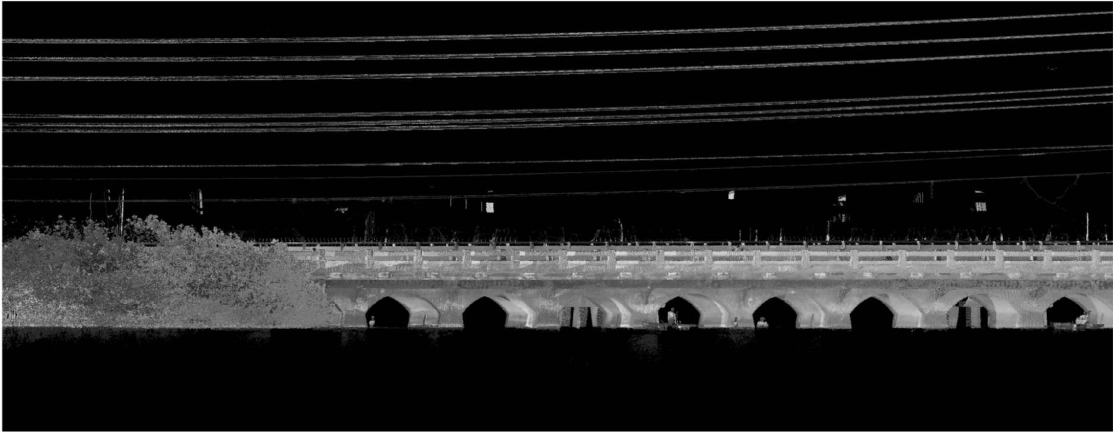
EXISTING ELEVATION VIEW OF SPAN NO(S). 1 THRU 12 (LIDAR SCAN-OCEAN SIDE)
