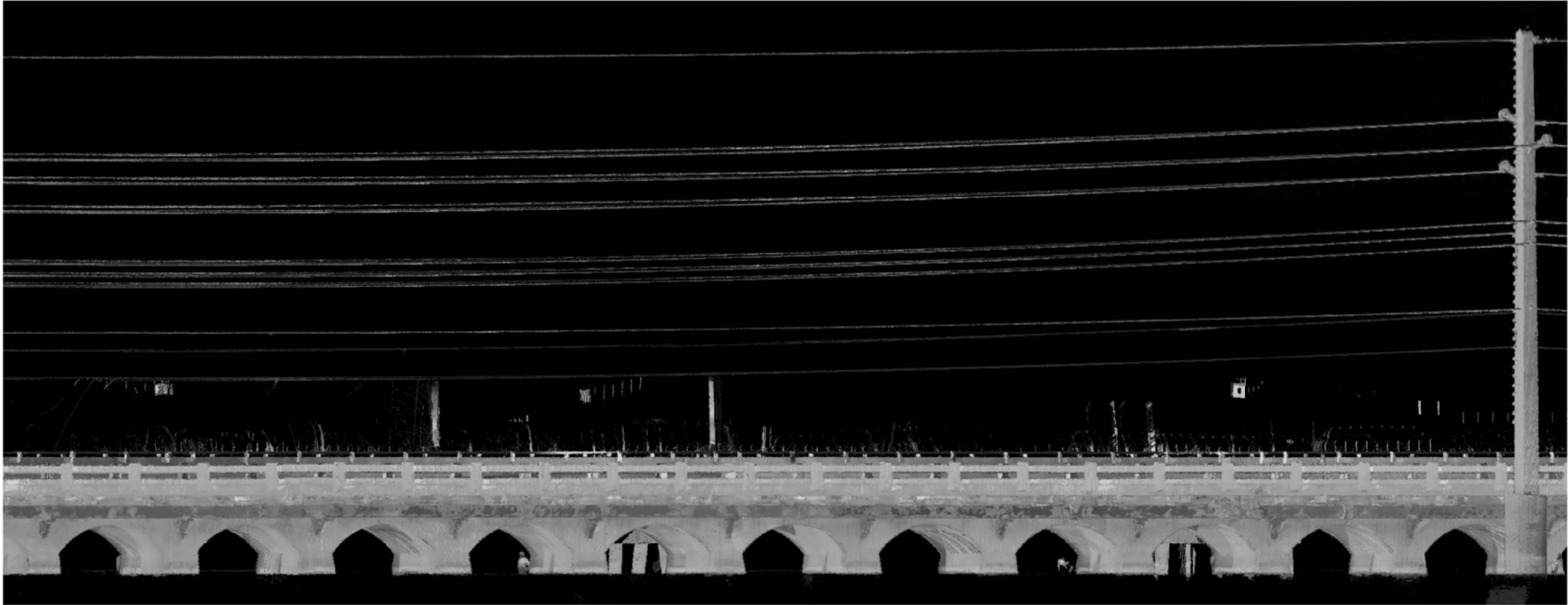
EXISTING ELEVATION VIEW OF SPAN NO(S). 61 THRU 72 (LIDAR SCAN-OCEAN SIDE)
