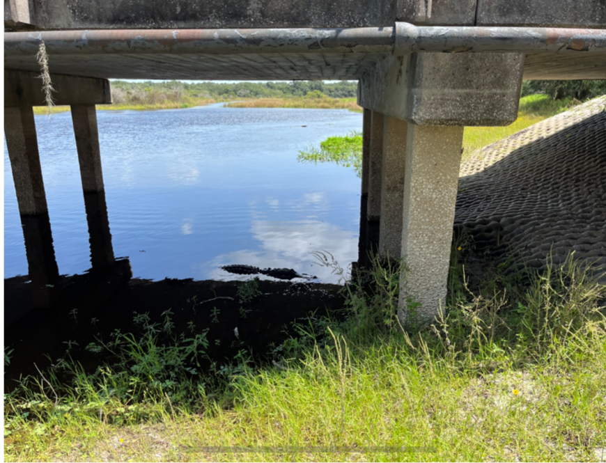
Figure 11 – View of the bridge's bent and piles.
