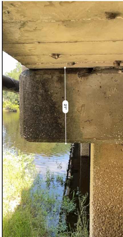
Figure 10 – Bent dimensions
