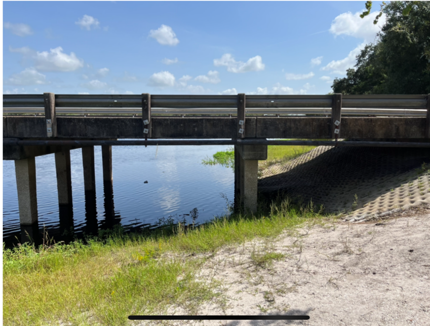
Figure 1 – Upstream section of abutment of the Myakka State Park bridge at East End Bent..
