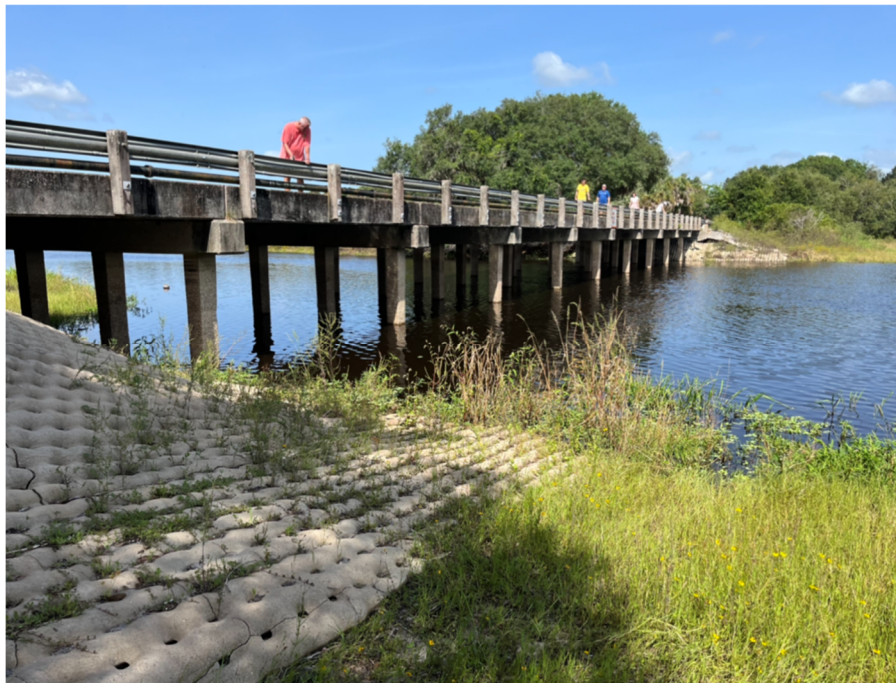
Figure 4 - View of the downstream section of the Myakka State Park bridge. East end bent in foreground
