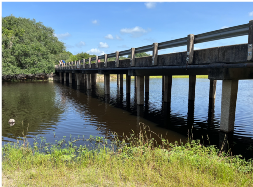
Figure 2 – View of the upstream section of the Myakka State Park bridge at East End Bent..
