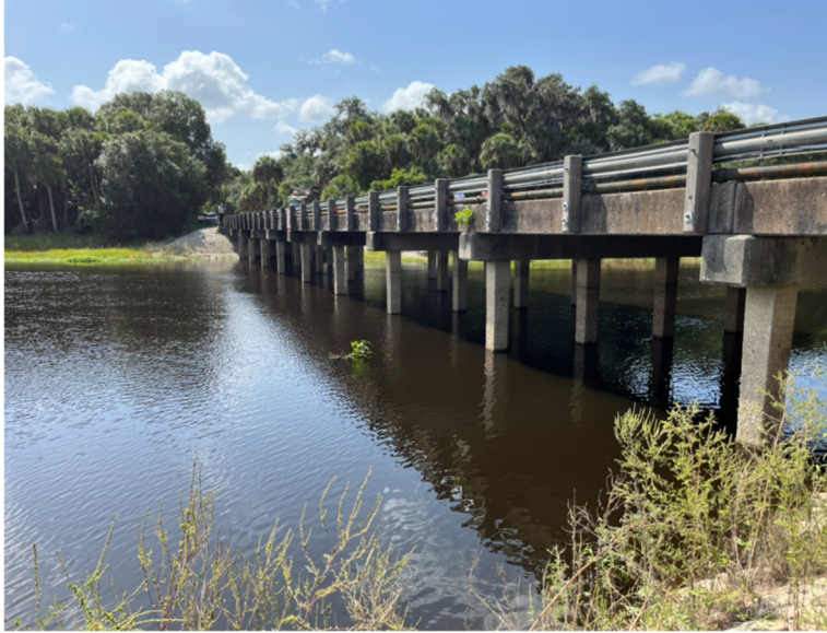
Figure 5 – Upstream view. West end bent in foreground.
