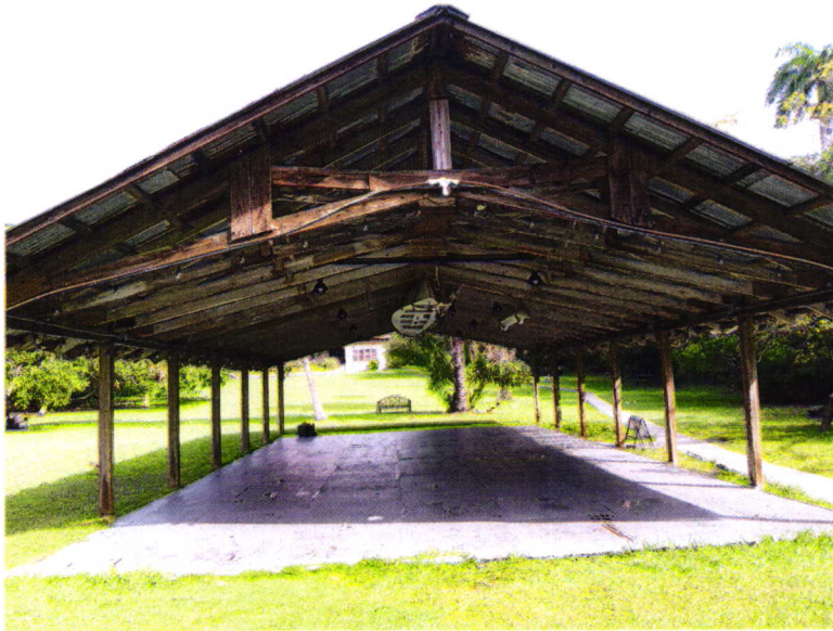
PHOTOGRAPH 1: Overview of pavilion
