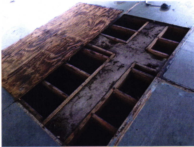
PHOTOGRAPH 7: Concrete beam under wood subfloor
