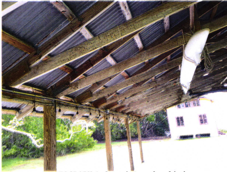
PHOTOGRAPH 4: Second view of roof deck
