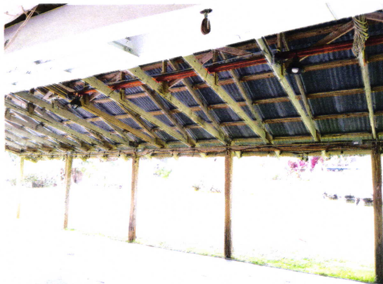
PHOTOGRAPH 3: Sheet metal deck above wood rafters
