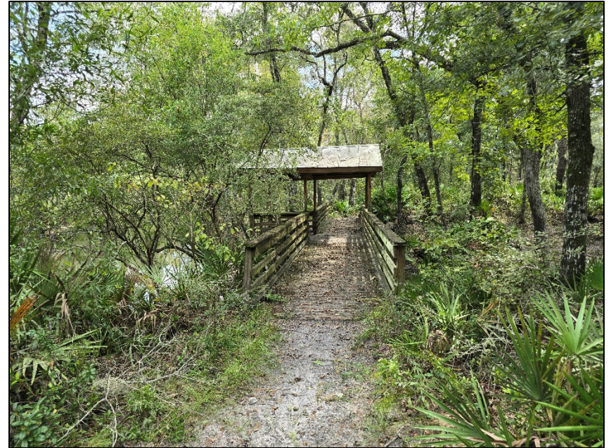
West side of Boardwalk 2.
