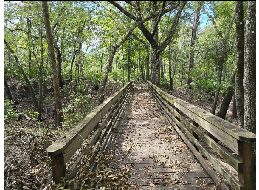
Boardwalk 5 existing structure.
