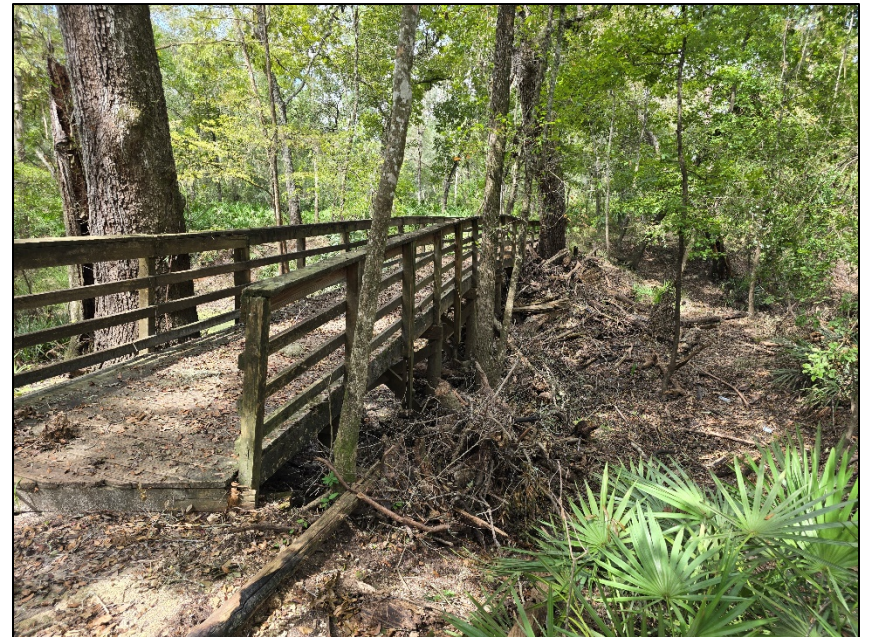
East side of Boardwalk 4.
