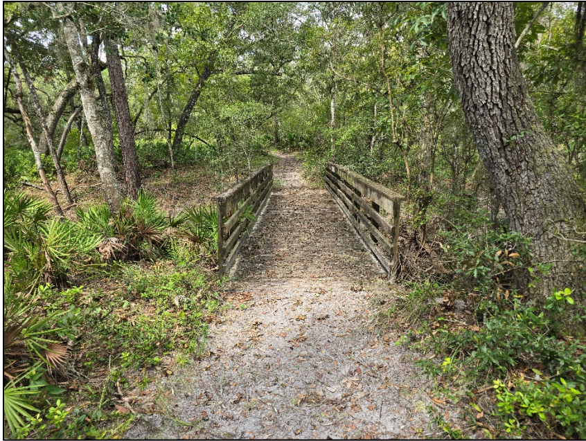
East side of Boardwalk 1.
