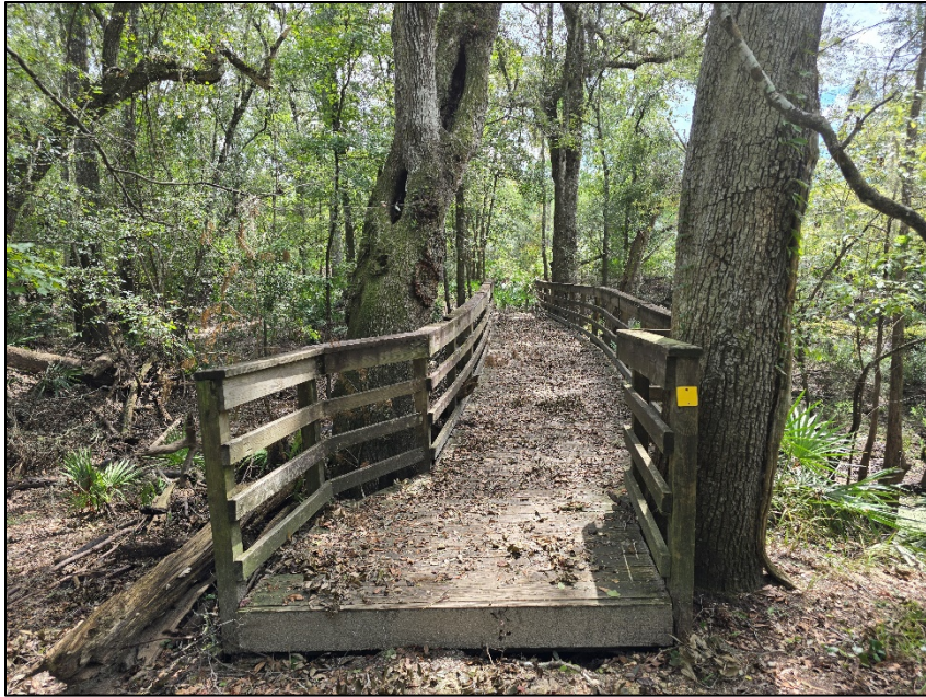
West side of Boardwalk 4.
