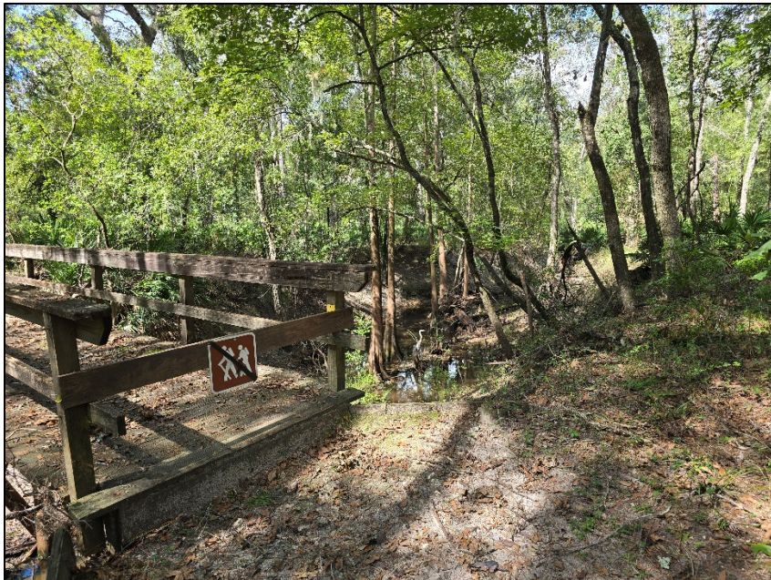
Boardwalk 6 adjacent community, facing northwest.
