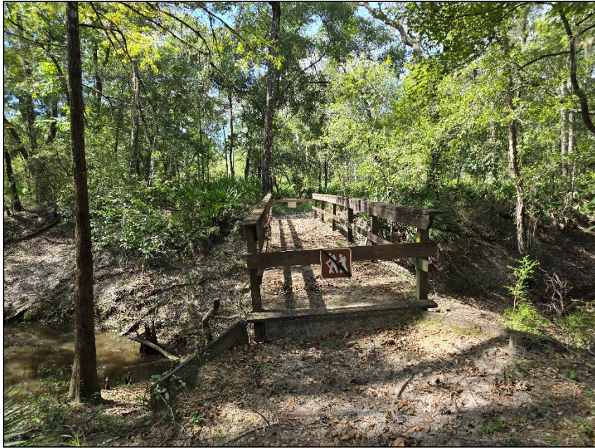
East side of Boardwalk 6.
