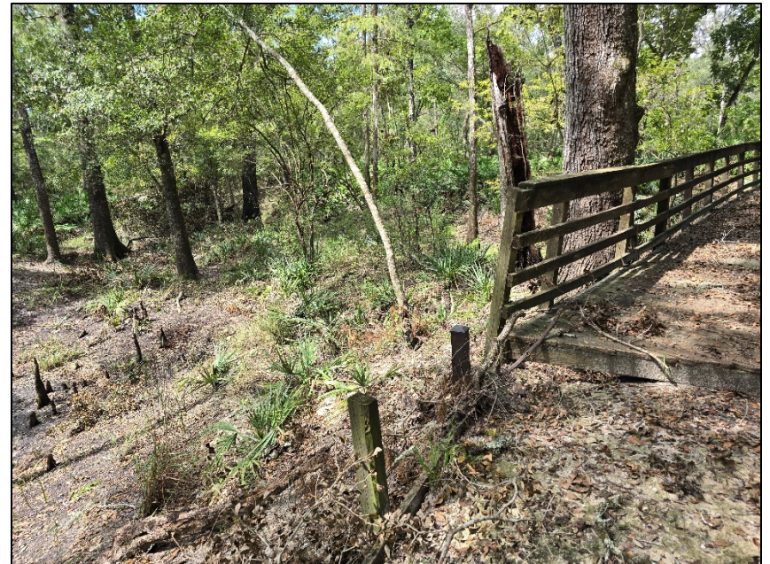
Wetland side of Boardwalk 4 from east end.
