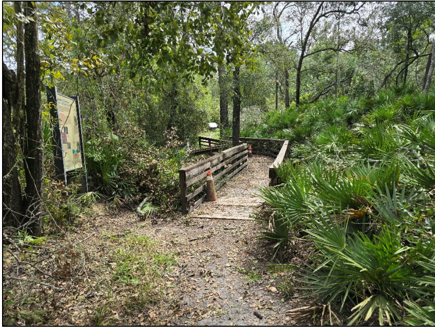
West side of Boardwalk 3.
