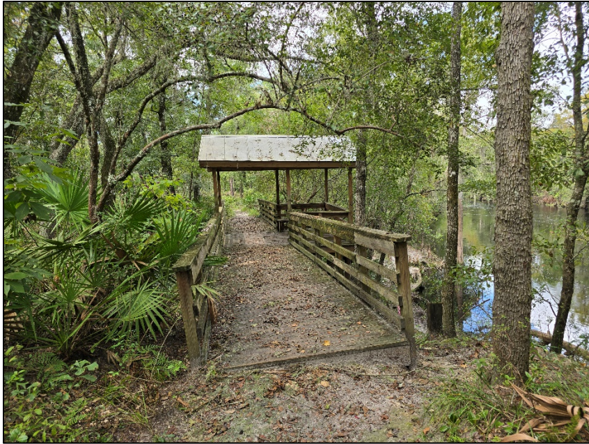
East side of Boardwalk 2.
