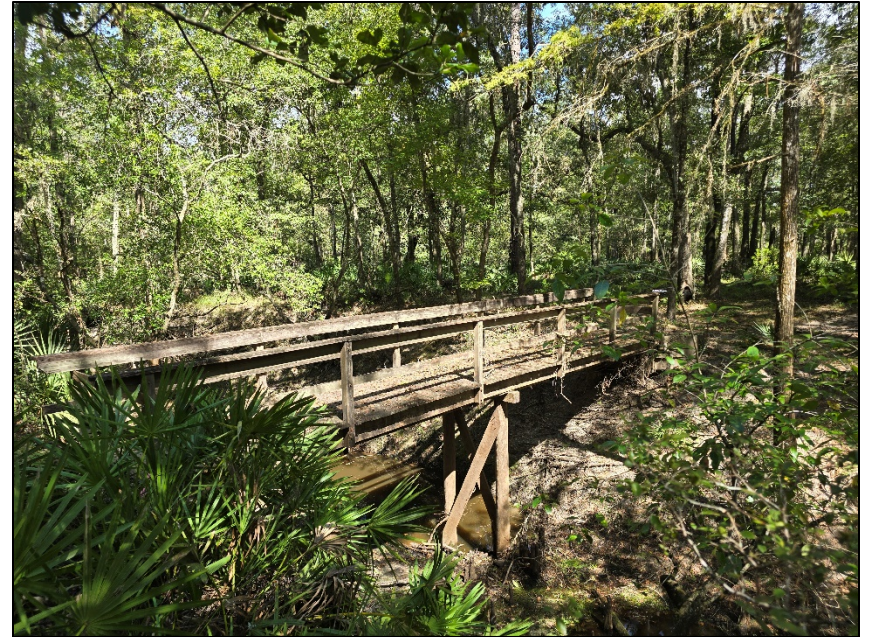
Boardwalk 6 viewed from southwest.
