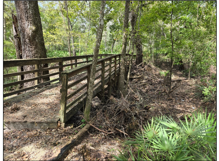
River side of Boardwalk 4 from east end.
