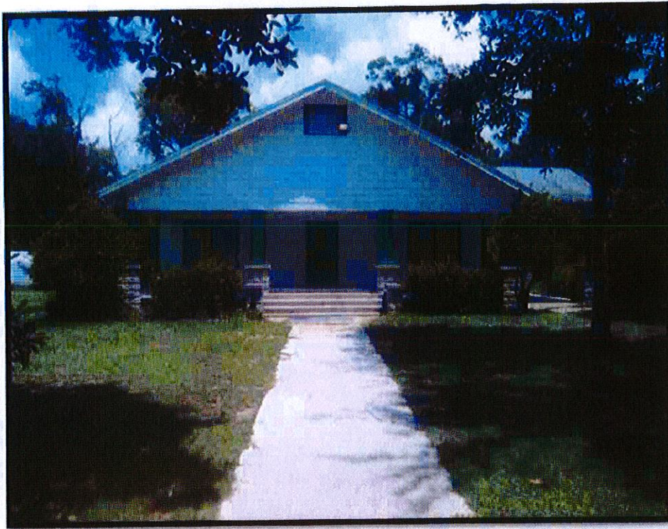
Figure 19. Photograph of the façade of 8CO1106 (Morrell House)
