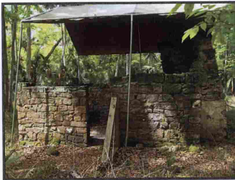
Figure 33. Current conditions of the wall elevations at the Addison's Blockhouse (8VO193) as noted during the GPS survey in April 2010
