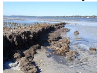
Fig. 3: Example of Erosion on Sawpit Island
