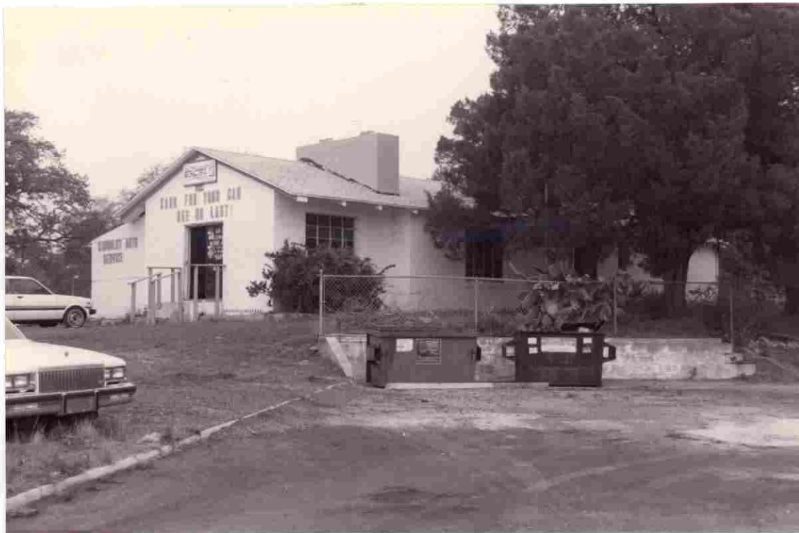
Figure 3. Photograph of Kingsley Auto Service (8HE390) facing west.
