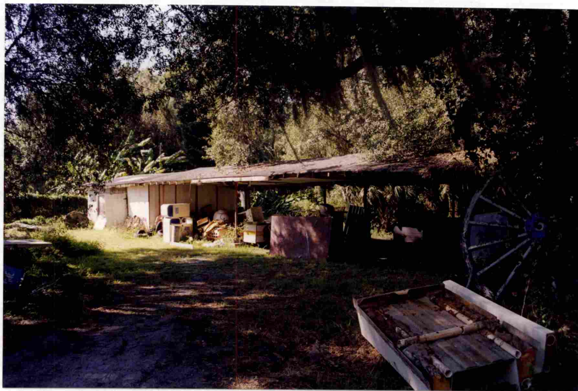
Photograph 9 Maintenance Building Roll 9871-1, #11; Facing northwest
