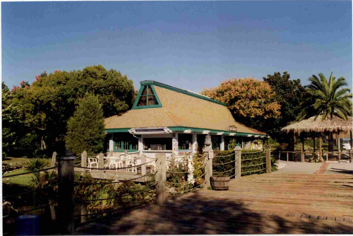
Photograph 4 Gift Locker Roll 9871-1, #1; Facing northwest
