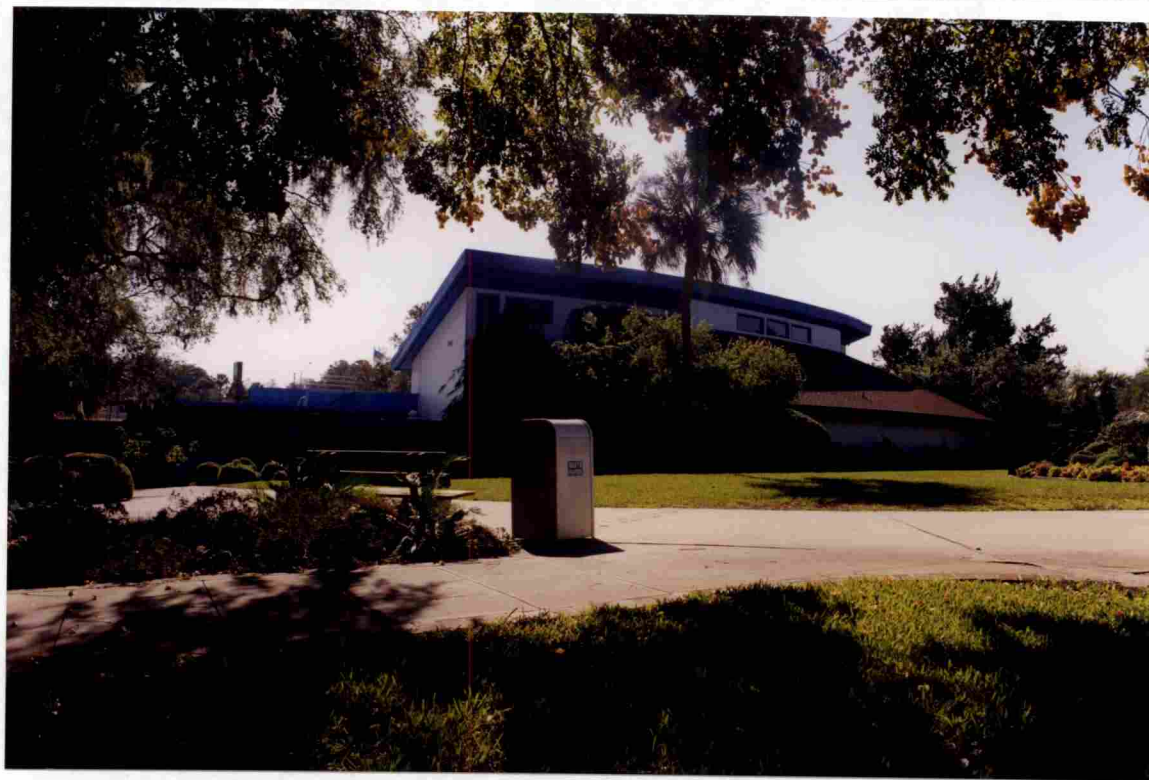
Photograph 11 Mermaid Theatre exterior Roll 9871-1, #6; Facing southwest
