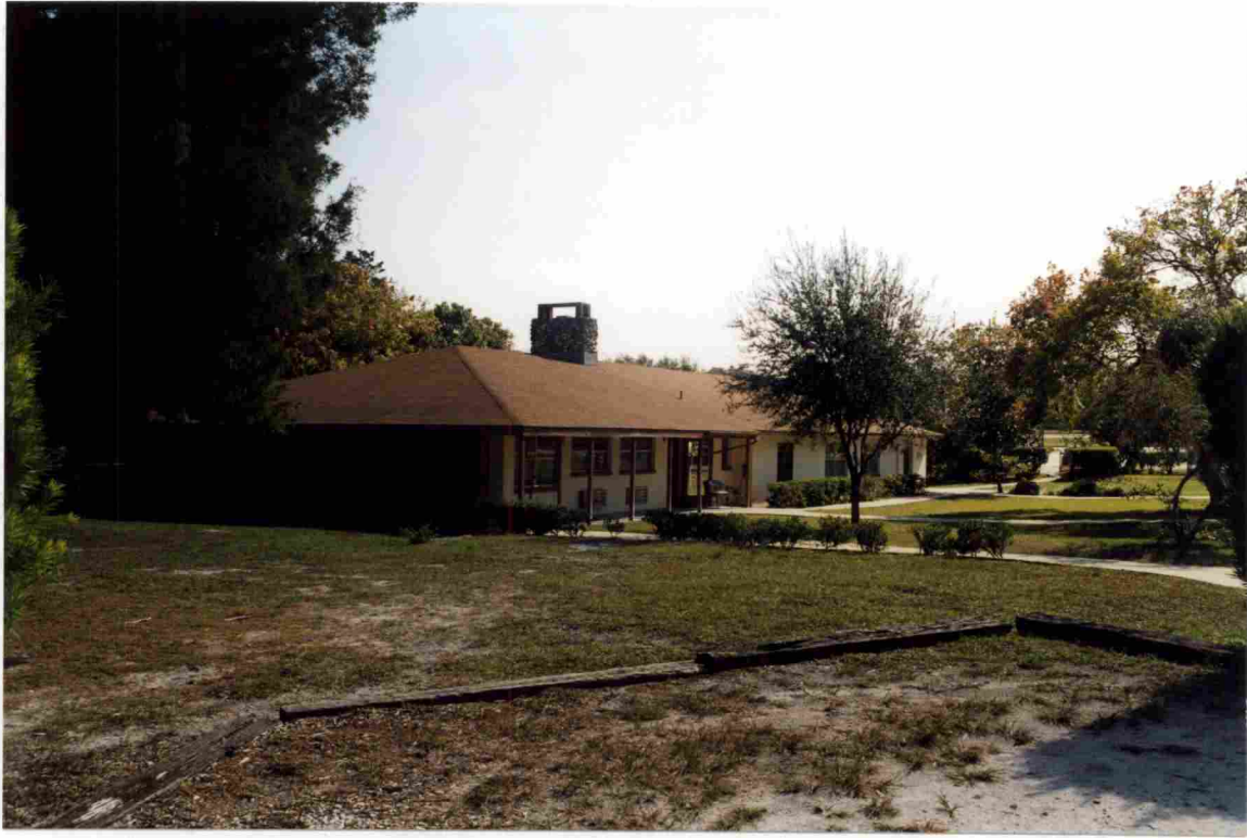
Photograph 8 Administration Building Roll 9871-1, #14; Facing southeast
