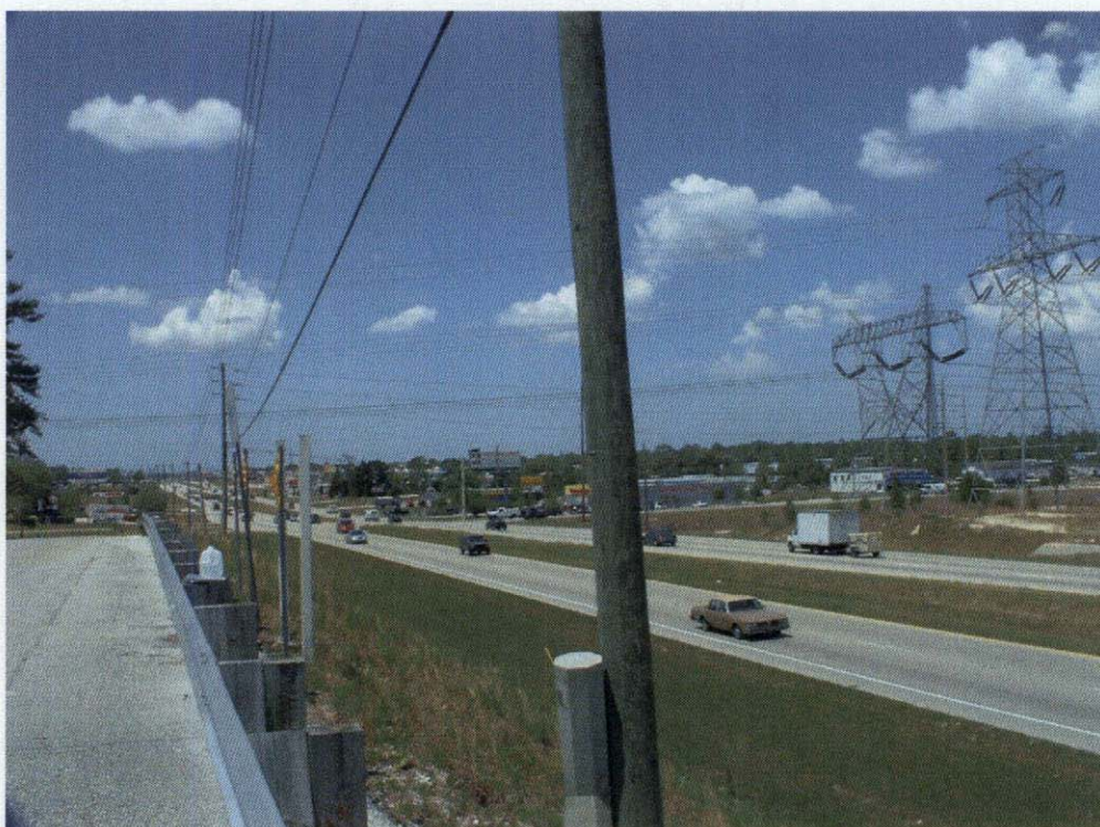
Photo 1.1. Looking Northwest Along S.R. 50.
