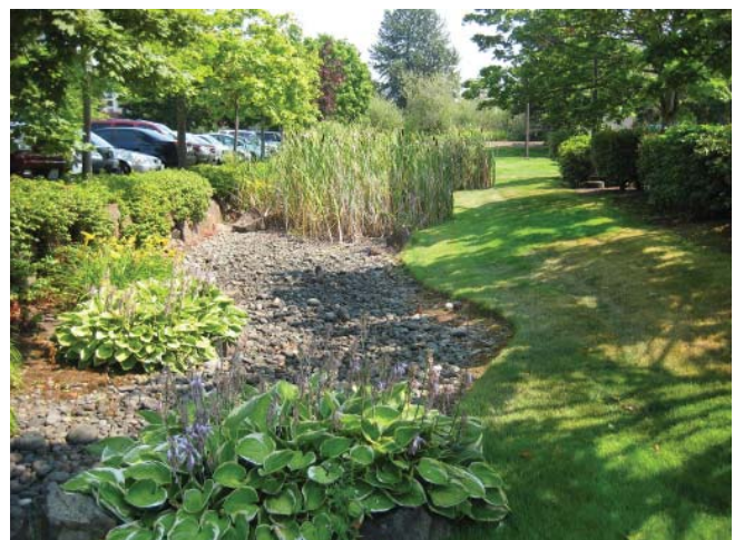
Bioswales, like the ones shown, are designed to capture and treat stormwater runoff. Native vegetation and design principles can be used to add color, texture, and form to bioretention features. (top: Cornell Plantations 2012, bottom: Pinehurst Seattle 2008)
