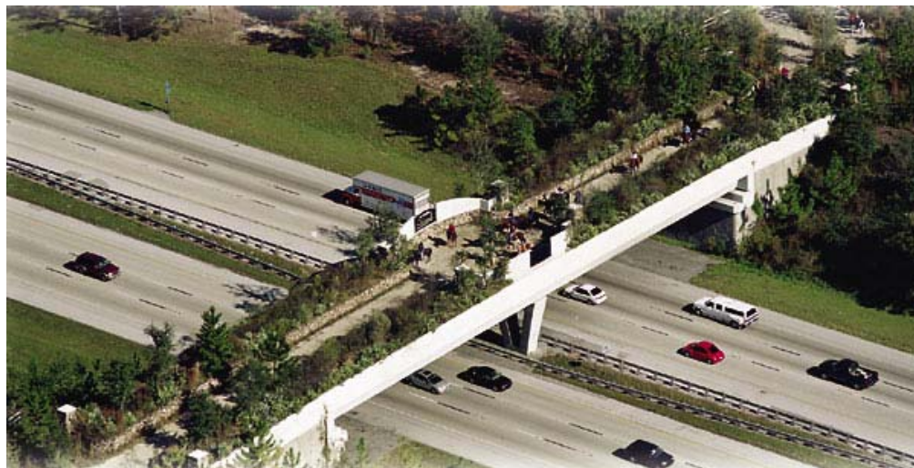
Cross Florida Greenway Land Bridge, Marion County
