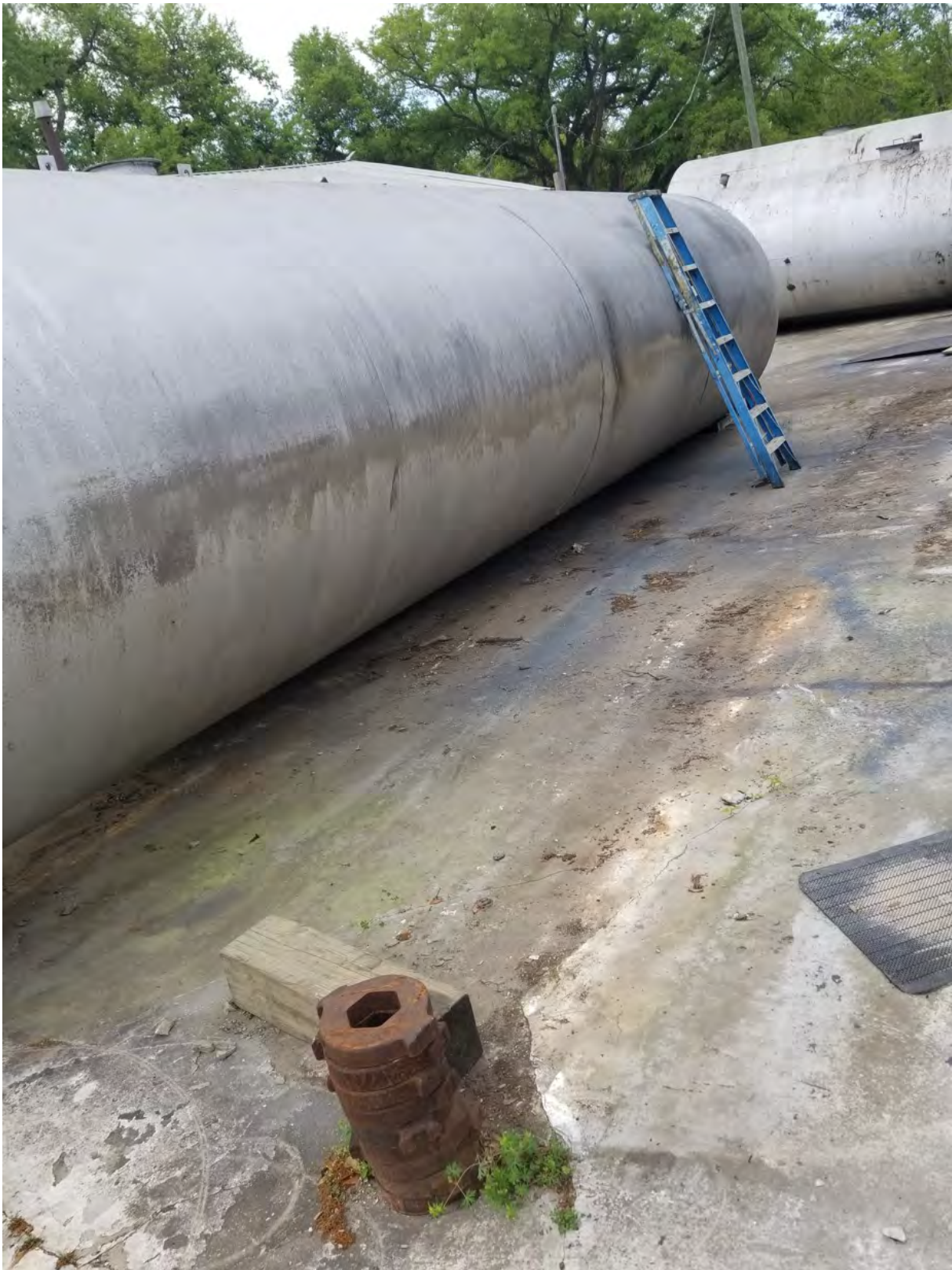
Figure 6: Containment area where tank #1 was previously located
