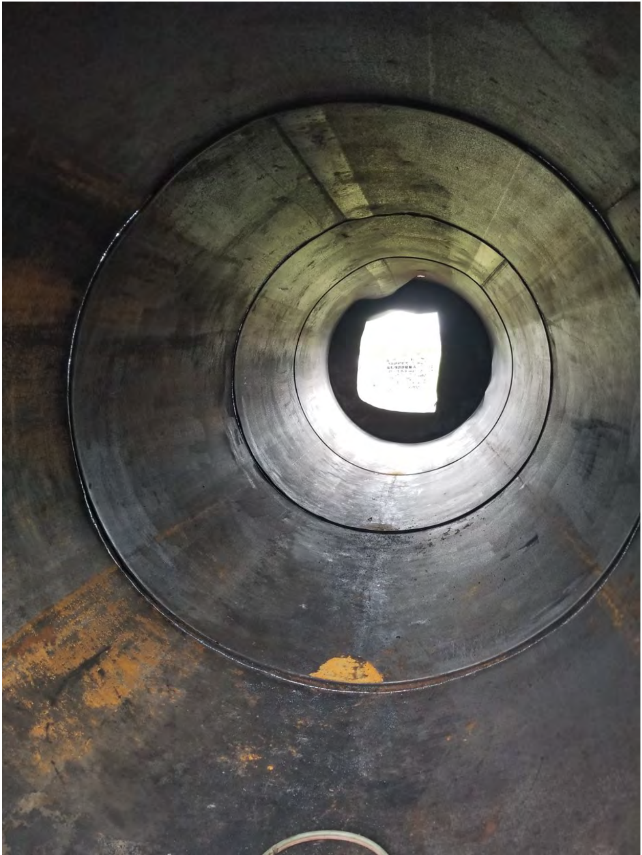
Figure 8:Interior of Tank #2
