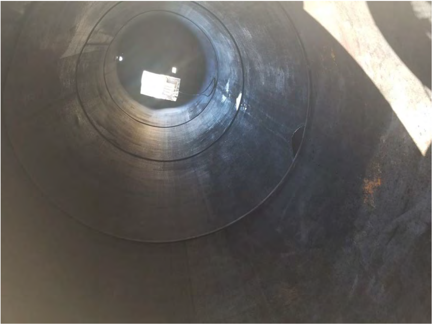
Figure 1: Inside Tank 1 after steam clean
