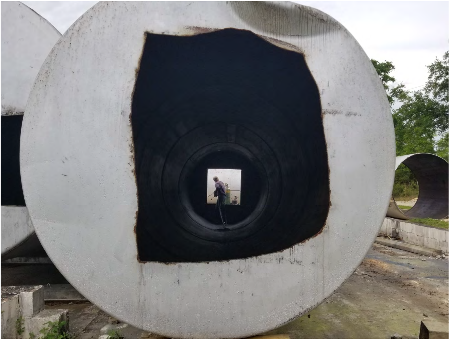
Figure 7: Process of cutting Tank #2
