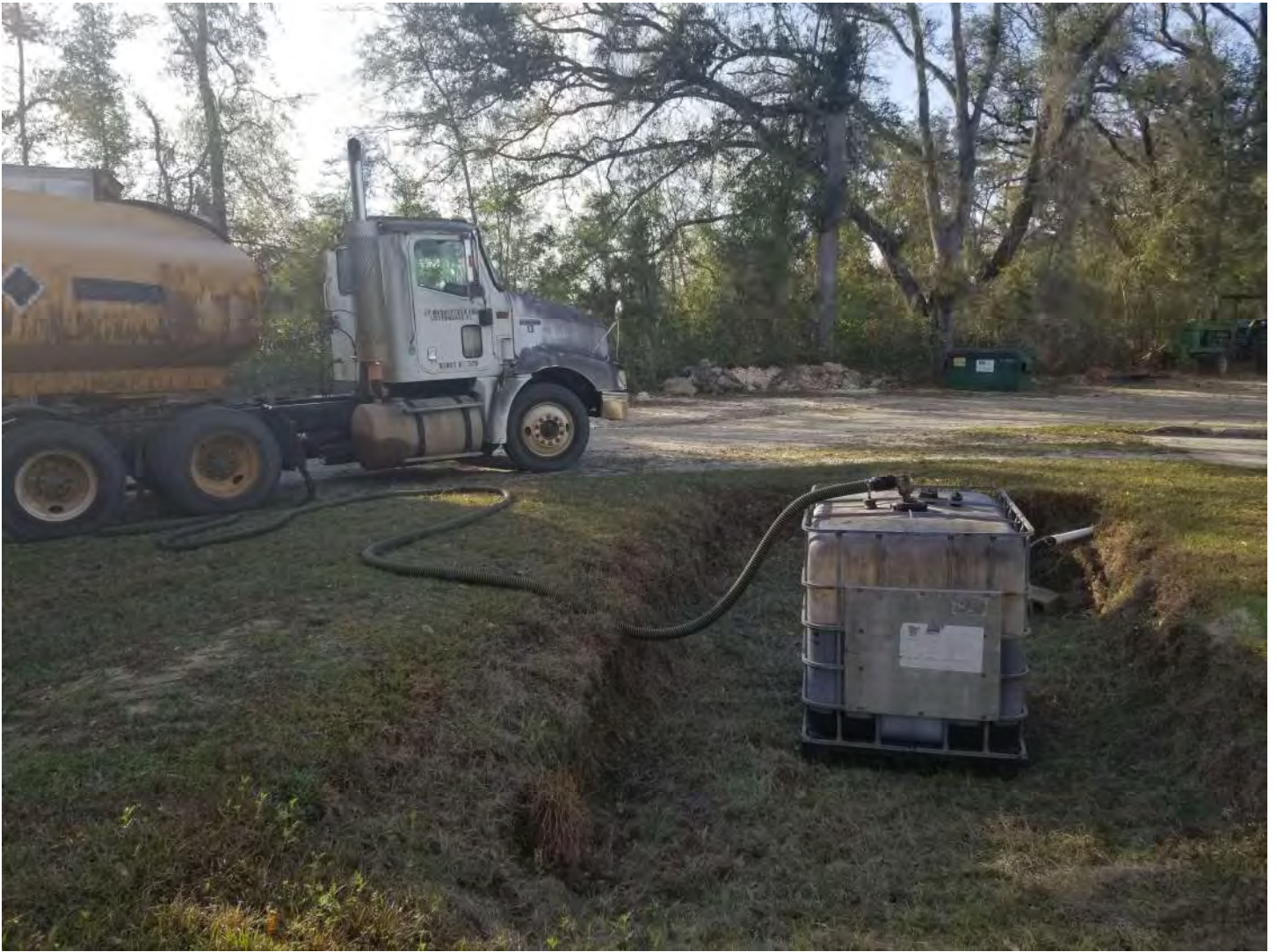
Figure 14: Tanker and pump
