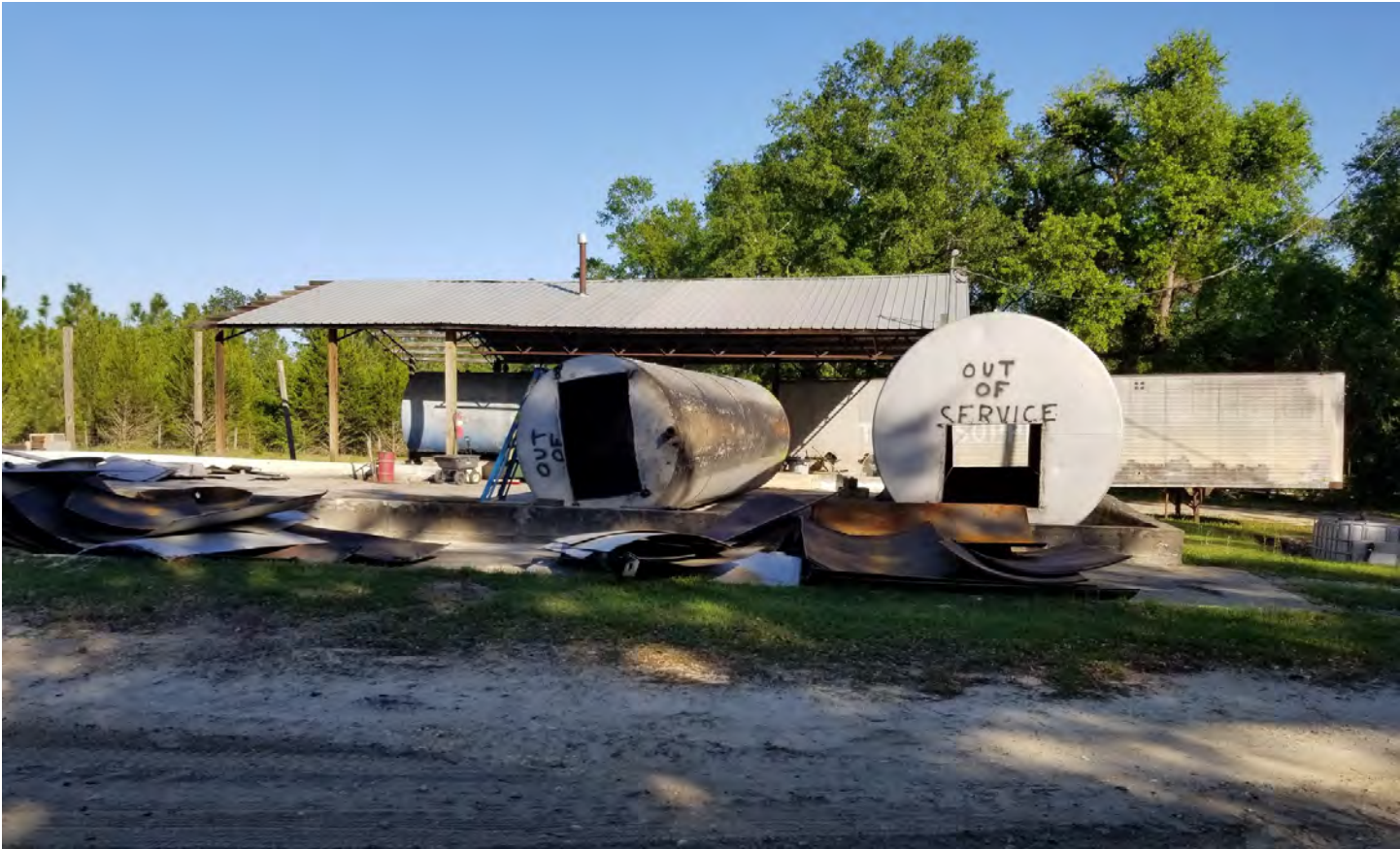
Figure 2: Tank #3 and Tank #4
