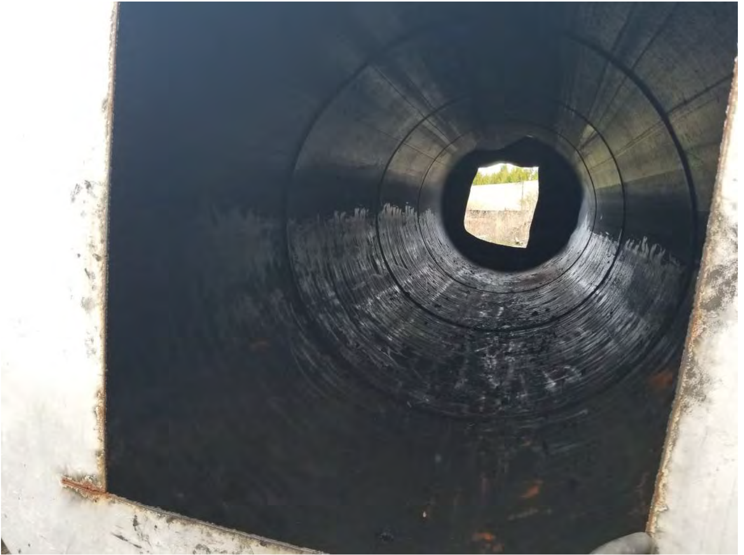
Figure 3: Inside of Tank 2
