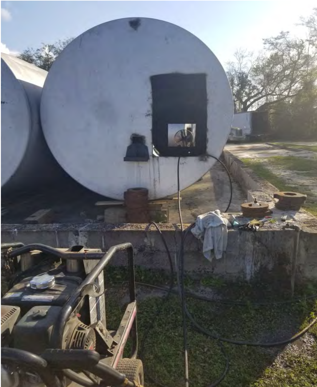
Figure 5: Tank 1 with steam cleaner setup
