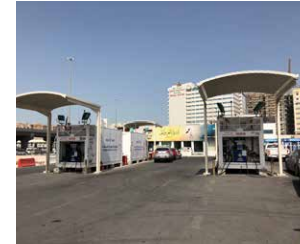
MODULAR FUEL STATION, QATAR
