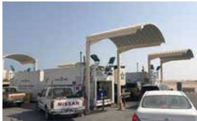
Modular Service Station Qatar
