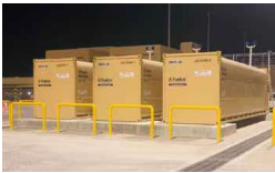
ROYAL OMAN NAVY - Fuelco supplied 3 x LTKO68 40ft UL142 Tanks for Vessel Refuelling
