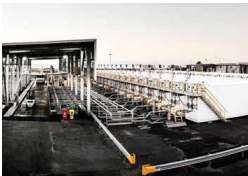
CASTROL BP - 43 x Logitank LSB110 self bunded tanks, totalling 1.24 million USG of storage for 16 lubricant product
