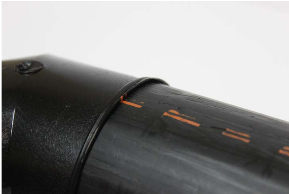
Close up of molded fitting to pipe weld, fitting bead remains slightly rounded, pipe bead has slight straight edge, due to processing differences of injection molded fitting versus extruded pipe. Bead height remains the same approx. \frac{3}{32} "
