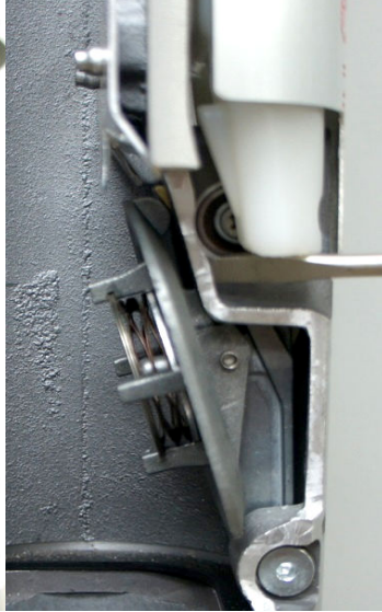
Primary float (shown raised - releasing the flapper valve)
