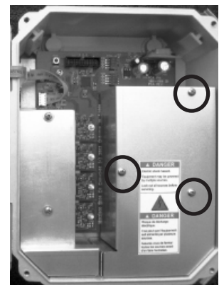
Figure 8 - Installing the Facilities Cover
