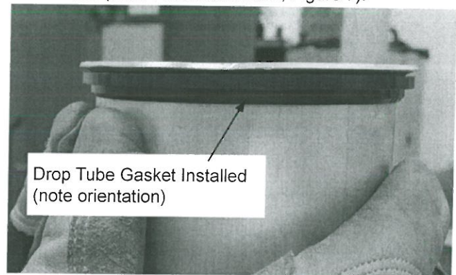
Figure 7: Drop Tube Gasket Installed
