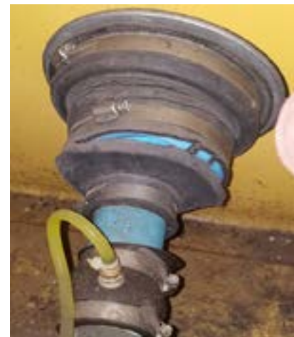
This repair would require IRF FL4.5
