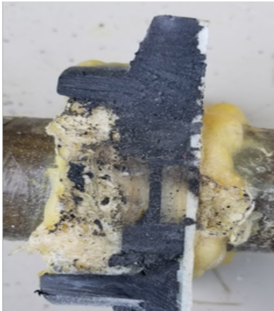
Icon SplitRepair Rigid Bonded Fitting Photo #10
