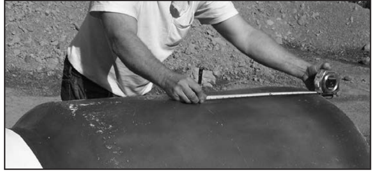
Figure 12 - Marking the Sump for Cutting
