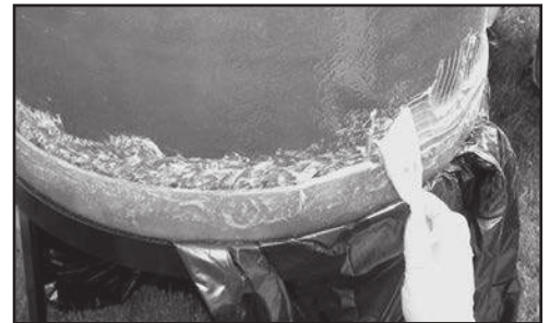
Figure 4 - Applying Catalyzed Putty
