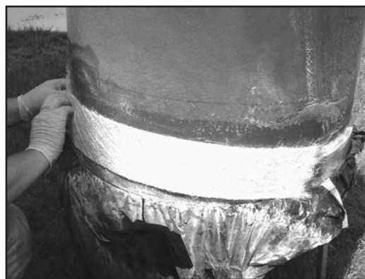
Figure 8 - Applying Mat
