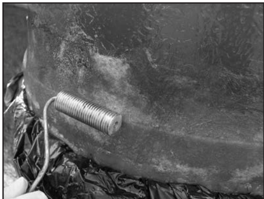
Figure 10 - Removing Air Bubbles
