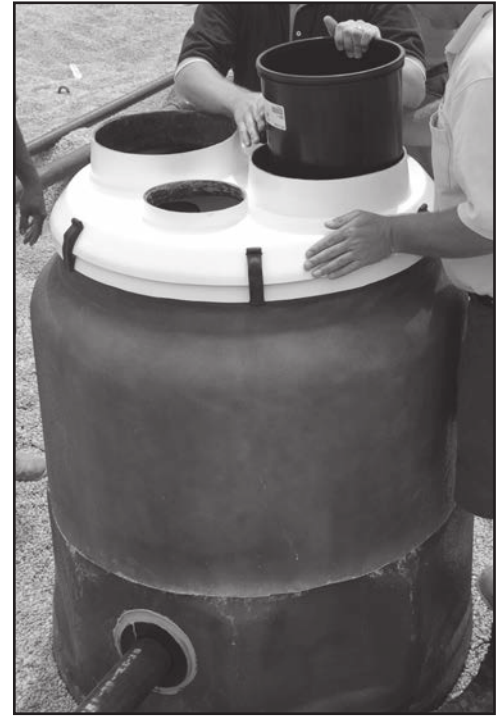
Figure 3 Aligning Multi-Port Sump Shield
