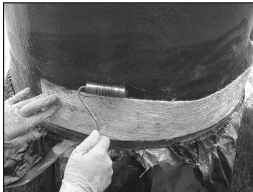
Figure 11 - Applying 2 nd Layer
