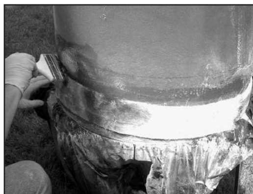
Figure 9 - Saturating with Resin
