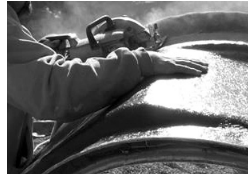
Figure 1 - Removing Bottom Ring
