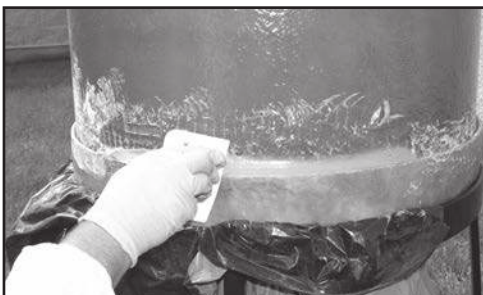
Figure 5 - Smoothing Catalyzed Putty
