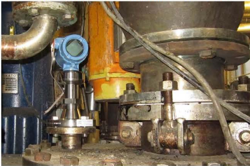
Figure 5. Rosemount 5408 Mounted on a Flange Intended for Tank Equipment
