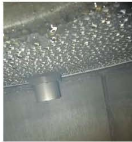
Figure 7. The End of the 2-in Rosemount 5408 Antenna
