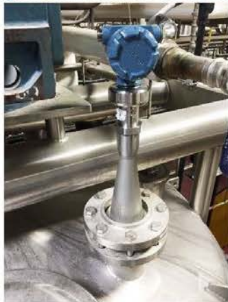
Figure 2. Rosemount 5408 Installed with a Rosemount 5402 Process Seal Antenna
