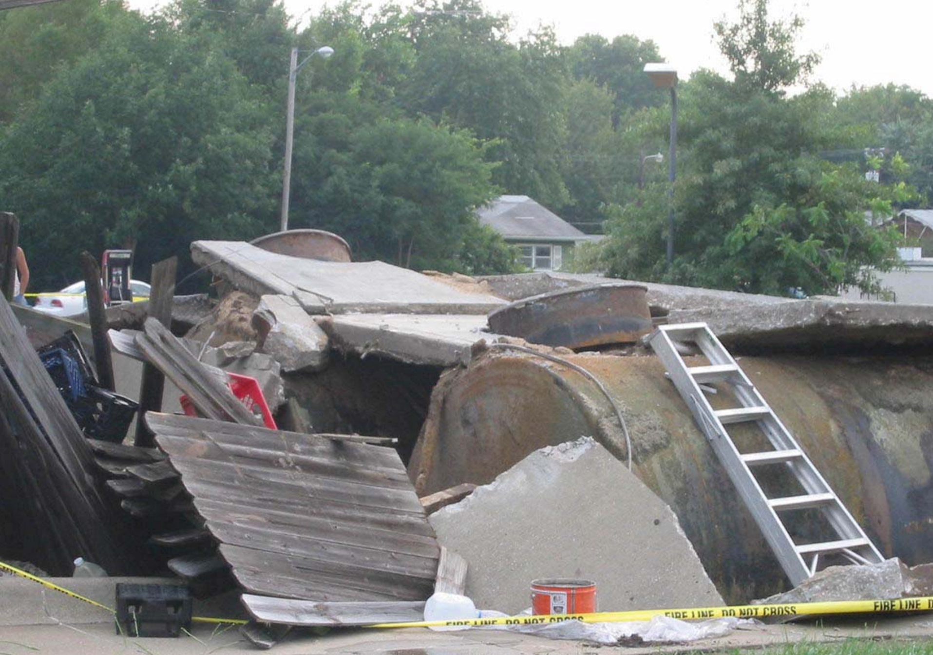
Improperly anchored USTs in Kansas
