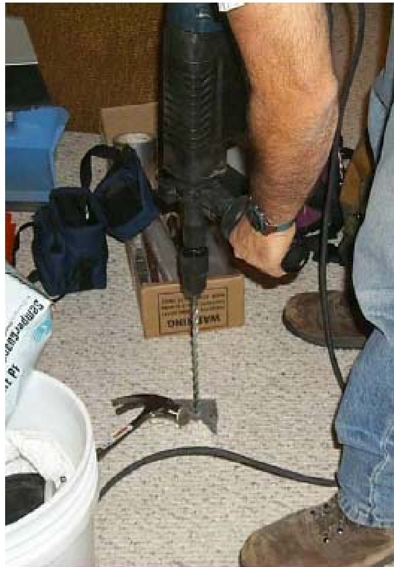
Figure 1. Drilling through a slab
