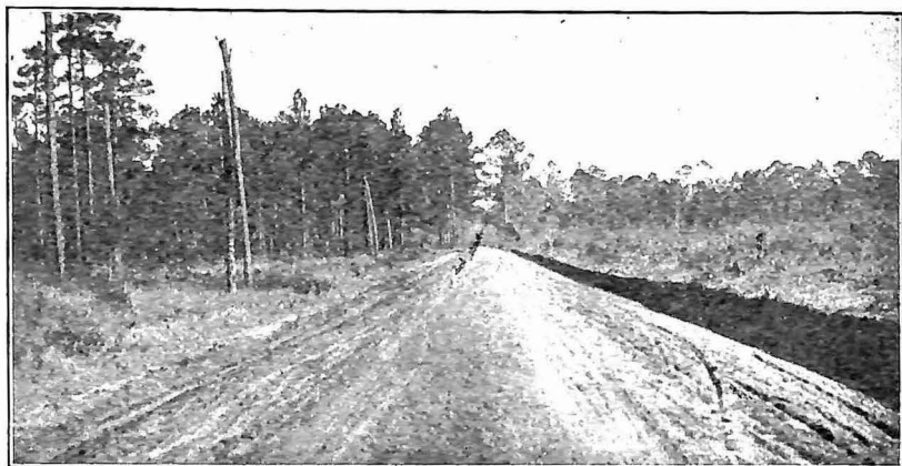
SAND-CLAY ROAD, ONE MILE NORTH OF VERNON, WASHINGTON COUNTY, FLORIDA.
