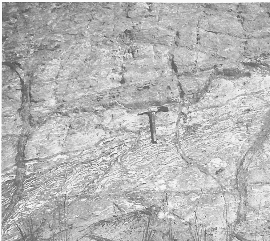
Figure 19. Roadcut showing clay laminae associated with very fine to coarse sands and also verticle joints filled with sandy clay.
