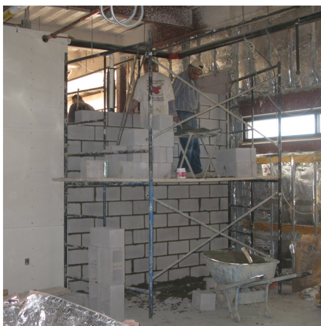
Concrete block going up for our specially-designed dye storage room.
