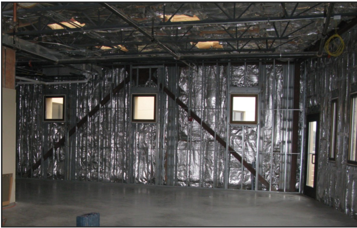
Steel studs start forming the walls in the NCKRI Library.
