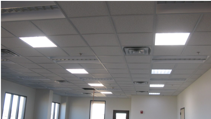
Skylights after the ceiling is finished. Look at all of the energy-saving natural light!
