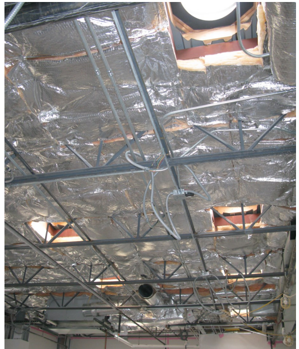
Skylights before installation of the ceiling.
