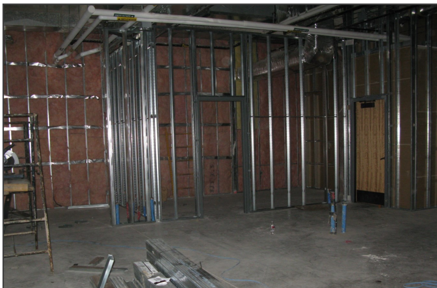
Walls starting to go up for the laboratory's storage room.
