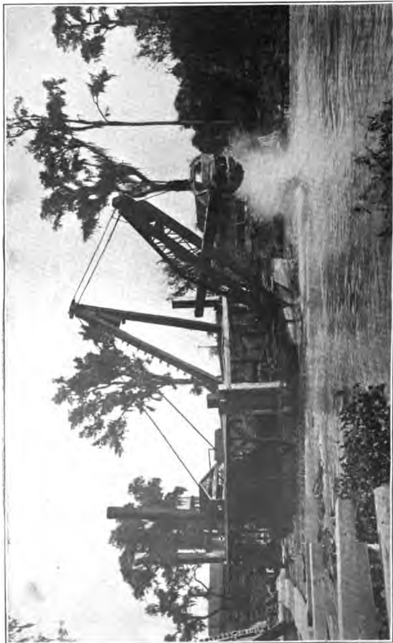
PHOSPHATE MINING IN FLORIDA BY FLOATING DREDGE, DUNELLON, FLA.
